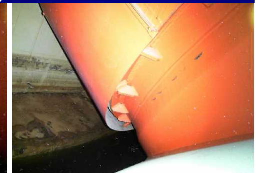
Bottom of venting pipe bellows cover
