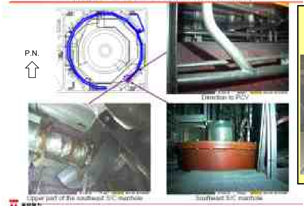
Result of the Investigation (Photos) 1/3
