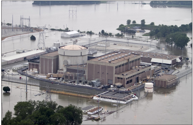
Fort Calhoun flooding event
