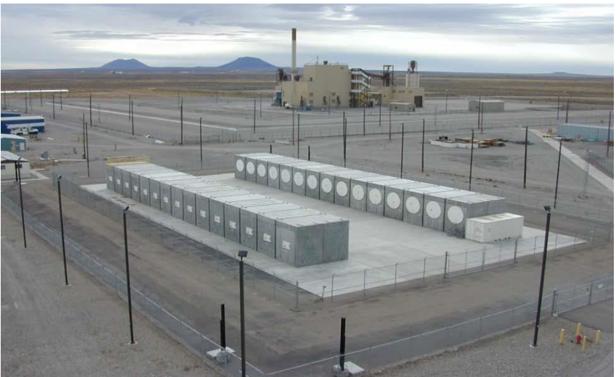
TMI-2 Independent Spent Fuel Storage Installation located at DOE's Idaho National Laboratory for interim storage of the TMI-2 core debris.
