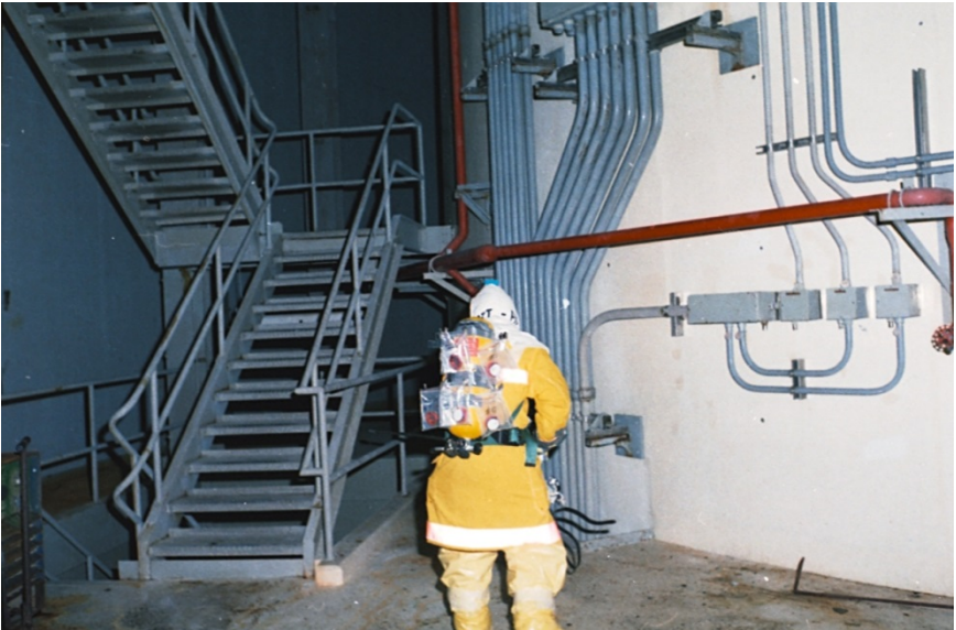
The first entry into the reactor building occurred on July 23, 1980 (shown). Heavy-duty outerwear provided protection from high-energy, low-penetration beta radiation.
