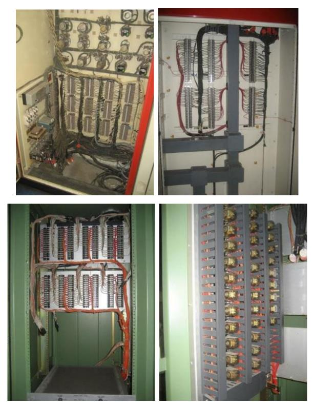
Figure C-28 Examples of "Low Fuel Loading" Sub-Category (1 of 2) Note that cables are neatly routed and tightly bundled and that there is a relatively low fuel loading given the overall enclosure volume.
