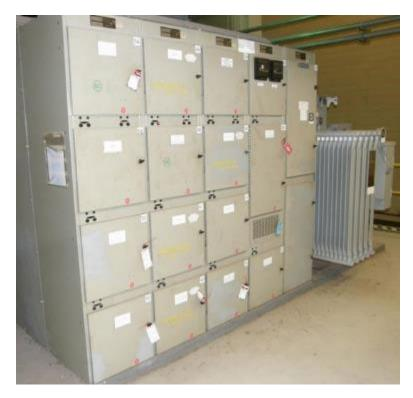
Figure C-7 Load Center (Left) with Oil-Cooled Transformer (Right)
