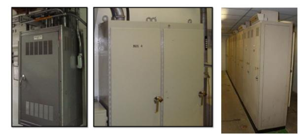
Figure C-21 Medium Enclosure (Approximately 0.6 m x 0.6 m x 2.1 m (2 ft. x 2 ft. x 7 ft.))
