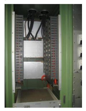
Figure 4-6 An Example of Non-Enclosed Wire-Ways That Would Not Qualify as Metal Enclosed Wire-Ways
