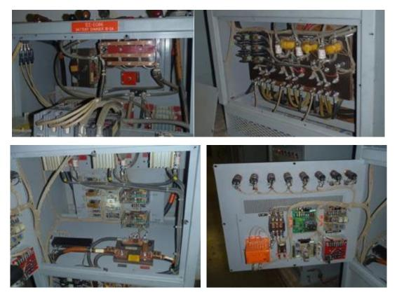
Figure C-14 Internal Views of Battery Chargers
