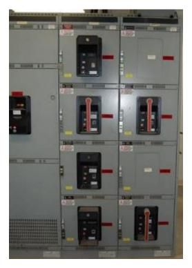
Figure C-9 Front View of Load Center (Low Voltage Switchgear)
