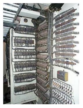
Figure C-20 Large Open Electrical Enclosure (Walkthrough Enclosure)
