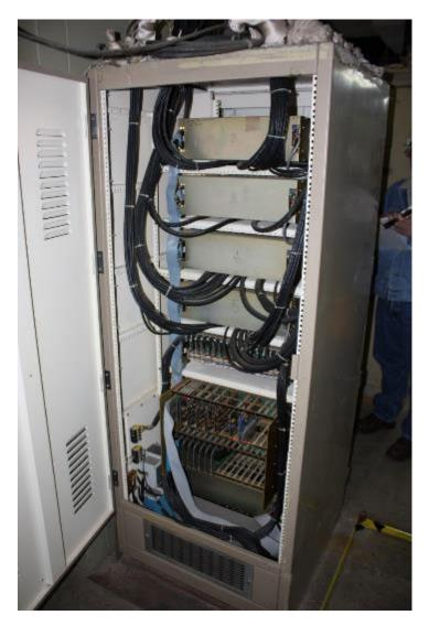
Figure C-29 Examples of "Low Fuel Loading" Sub-Category (2 of 2) Note that larger size cables are neatly routed and tightly bundled and that there is a relatively low fuel loading given the overall enclosure volume.
