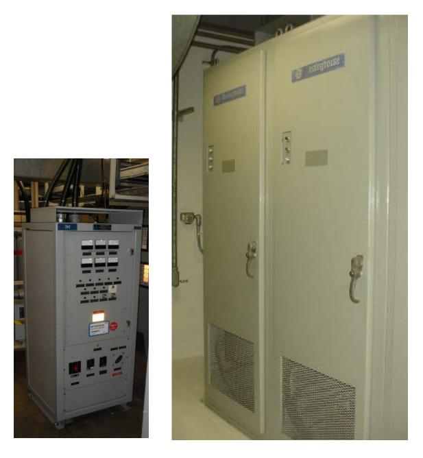
Figure 3-6 Examples of closed cabinets (a) fully closed cabinet and (b) closed with openings at the bottom
