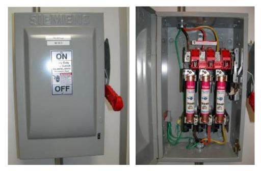
Figure C-23 Wall Mounted Low Voltage AC Fused Disconnect Switches
