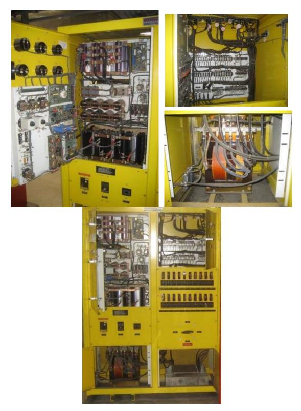
Figure C-16 Power Inverters – Internal Views
