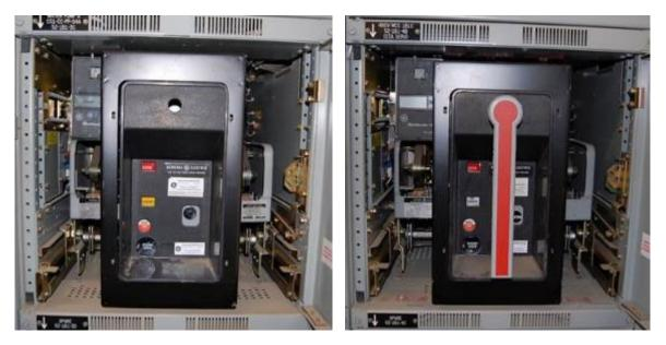
Figure C-10 Low Voltage Load Center Breaker
