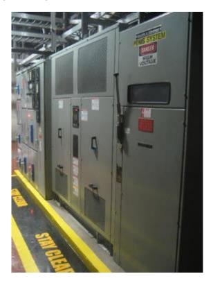
Figure C-5 Front View of Load Center (Disconnect Switch)
