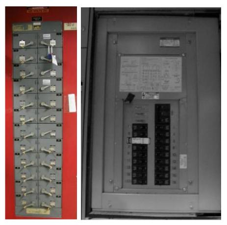
Figure C-24 125 VDC Distribution Panel (Left) and 120 VAC Distribution Panel (Right)
