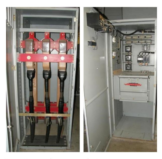
Figure 2-4. Photographs of the internal wiring of medium voltage switchgear.
