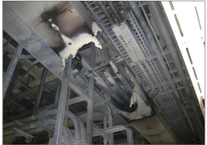
Figure 9.11 HEAF damage.
