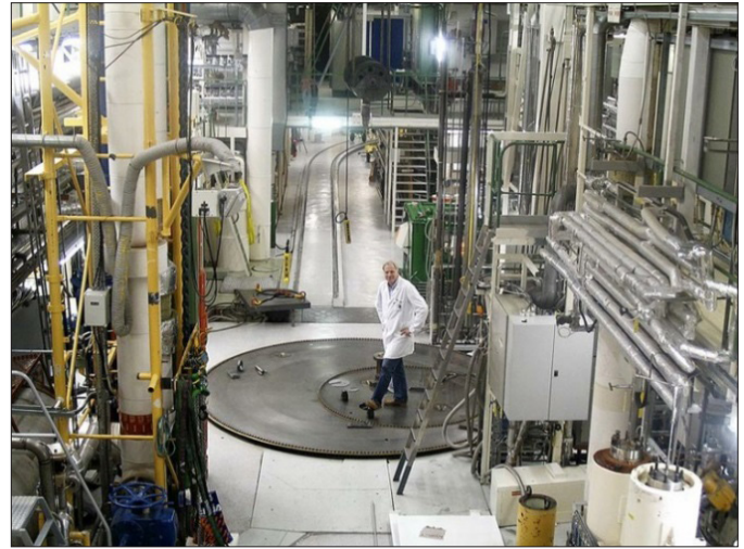
Figure 15.1 Halden boiling-water reactor.
