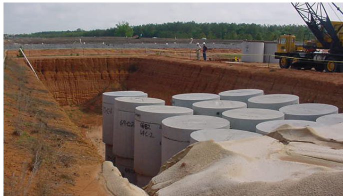
Low-level radioactive waste storage site.
