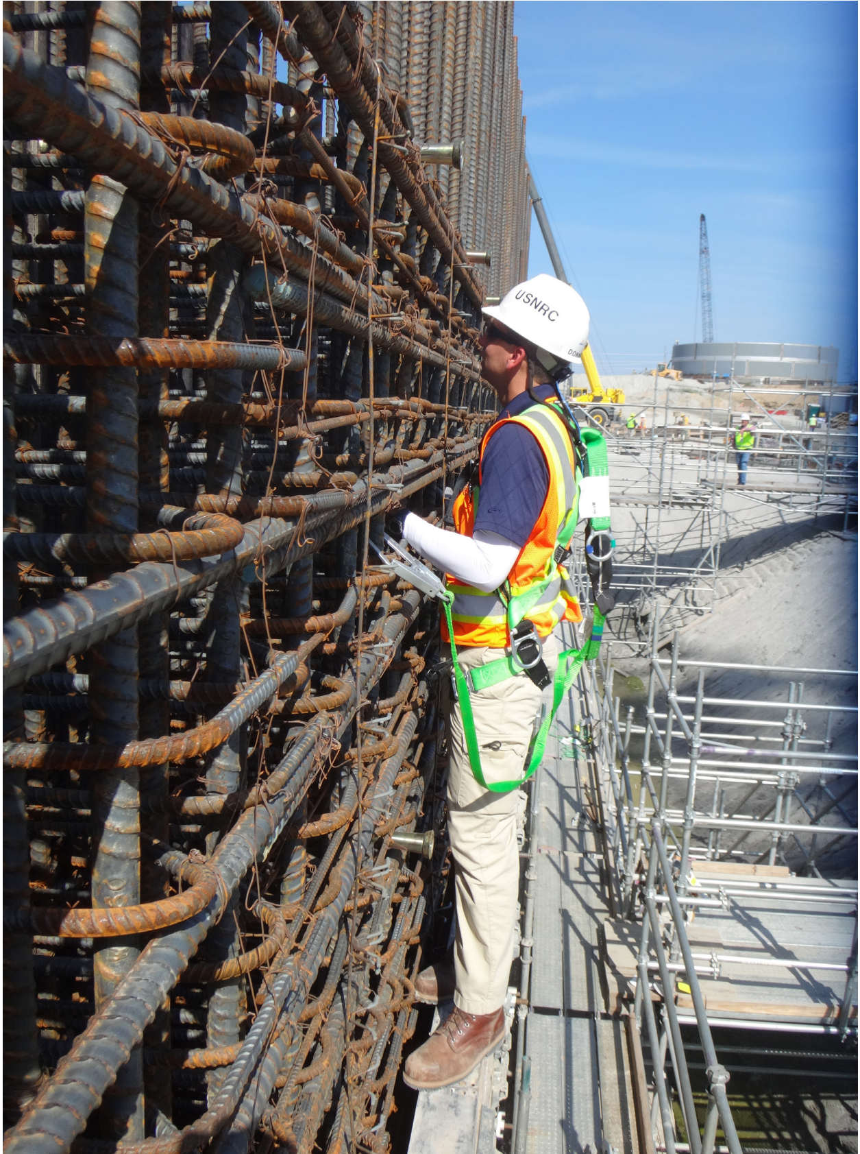
Inspection to construction at V.C. Summer nuclear power station.
