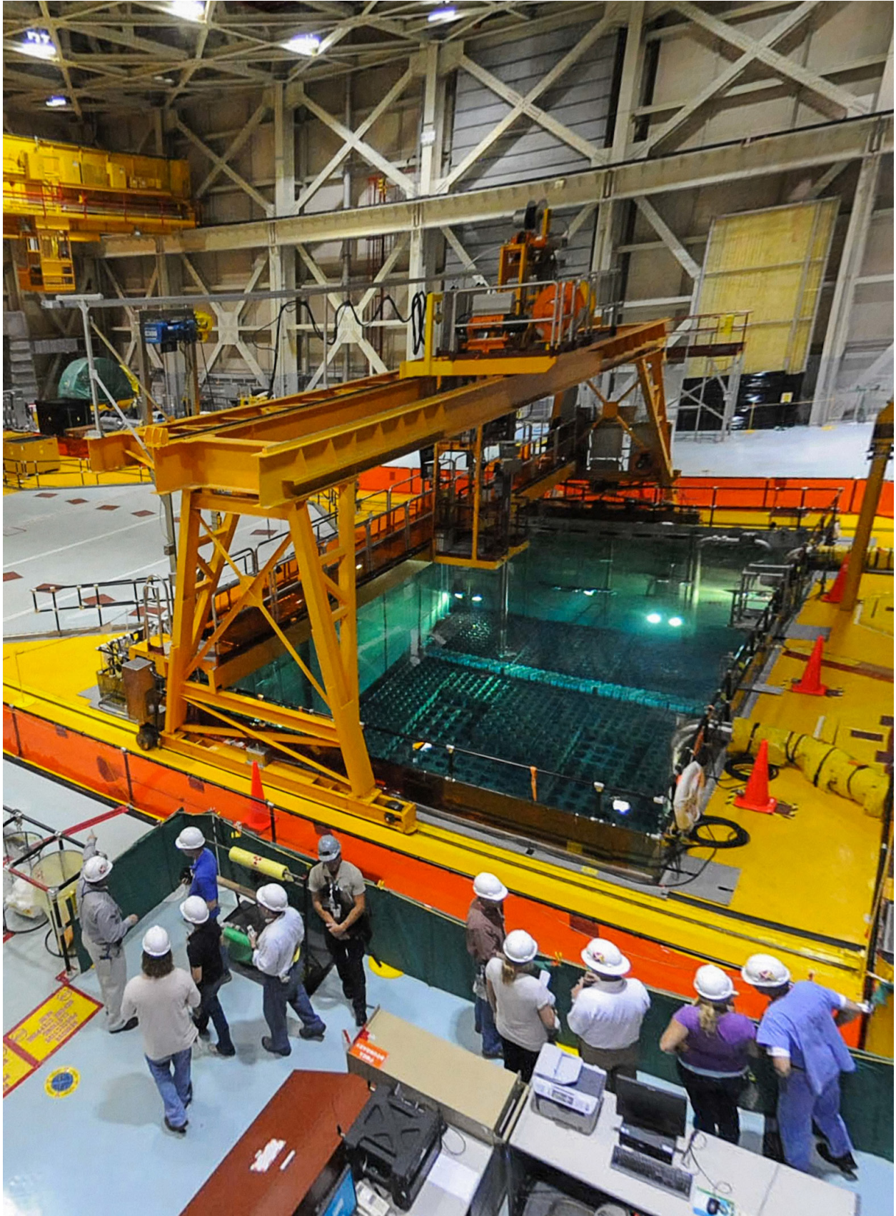
Spent fuel pool
