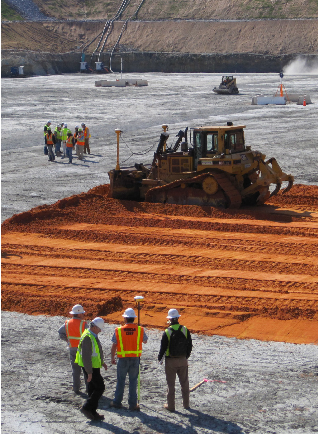
Backfill on Vogtle Unit 3. Photo courtesy of Southern Company
