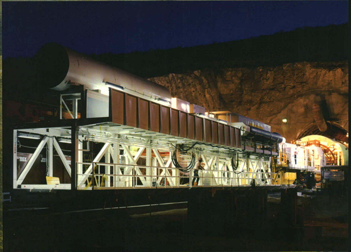
Tunnel Boring Machine at Yucca Mountain
