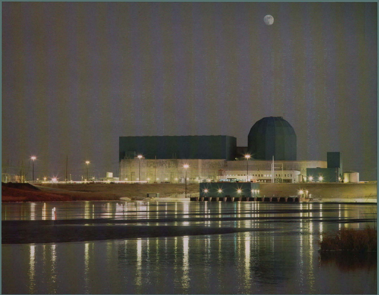
Clinton Nuclear Power Station
