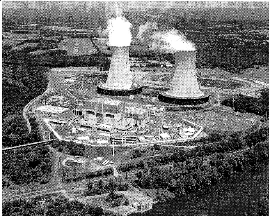
Limerick 1 and Limerick 2 Nuclear Power Reactors
