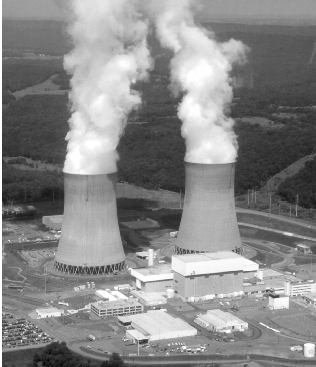
Susquehanna Steam Electric Station
