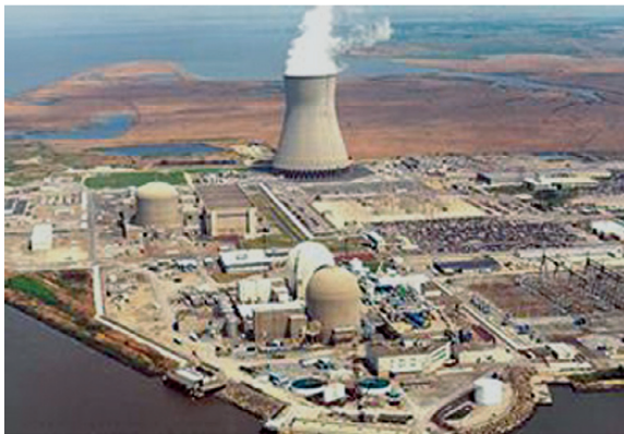
Hope Creek Nuclear Generating Station
