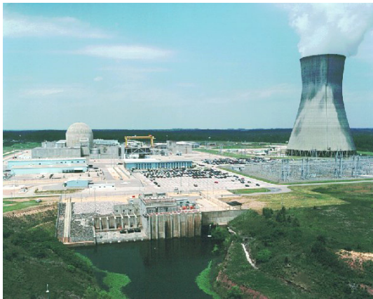
Shearon Harris Nuclear Power Plant
