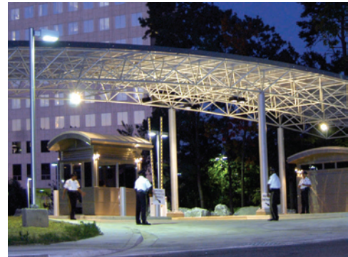
Guard station behind NRC Headquarters in Rockville, MD
