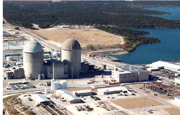
Comanche Peak Nuclear Power Plant
