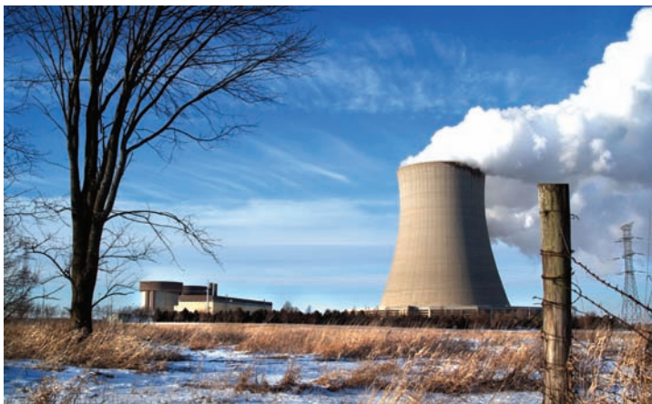
Byron nuclear power plant. Photo courtesy Exelon Nuclear
