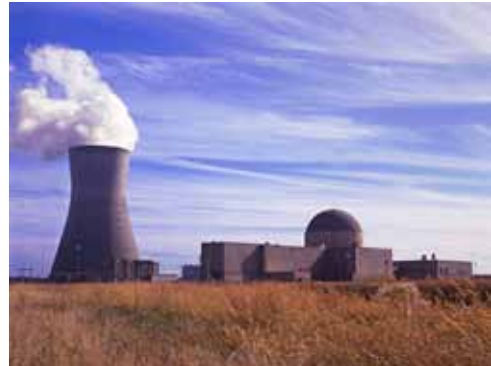
Shearon Harris Nuclear Power Plant. Photo Courtesy Progress Energy
