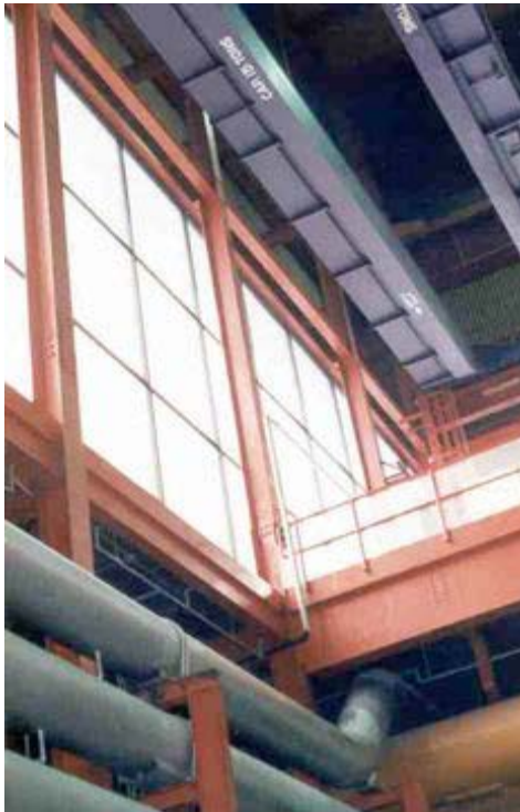
Figure C.8: Example of the Windows in Turbine Hall
