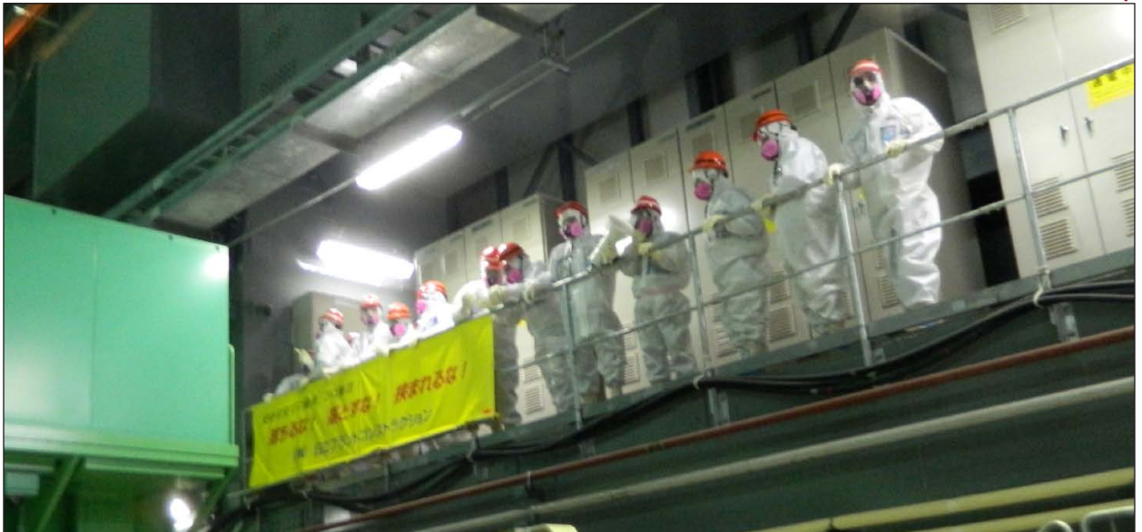
The NRC Team at the Fukushima Daiichi Unit 4 Spent Fuel Pool.
