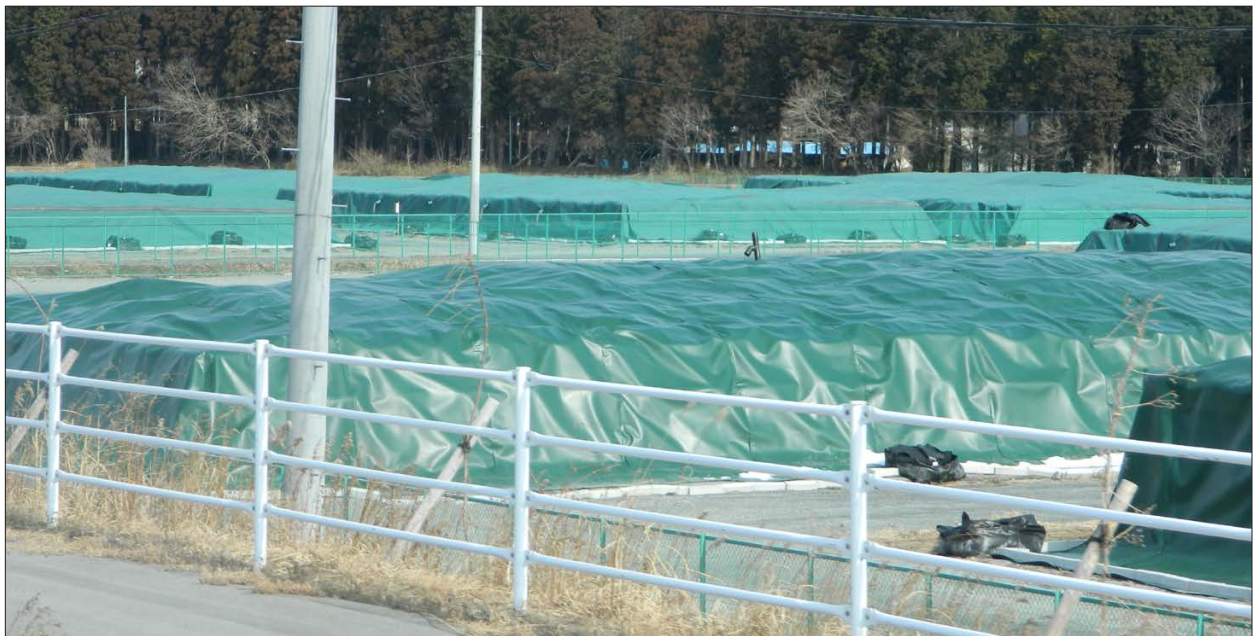
Contaminated waste storage in Fukushima Prefecture.
