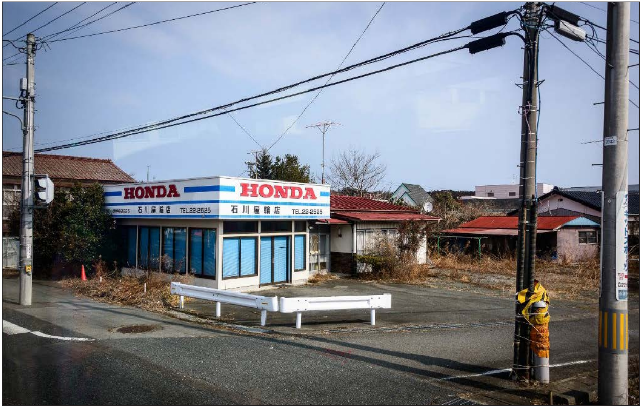
Abandoned stores in Tomioka, Fukushima Prefecture, Japan.
