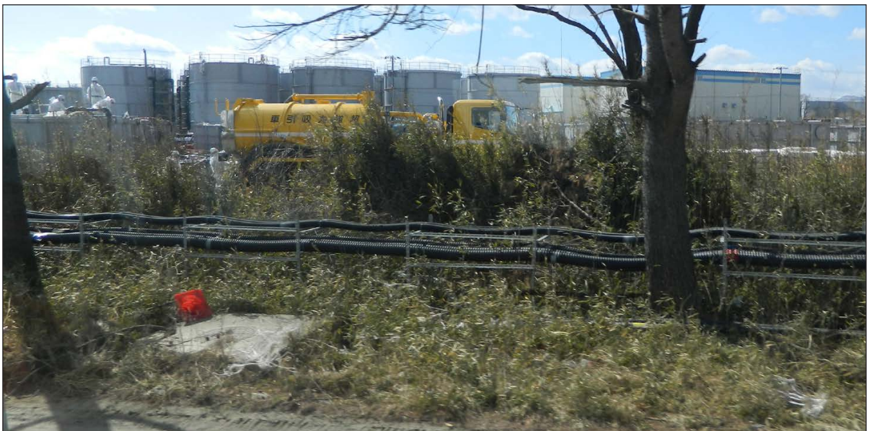
Water storage tanks at the Fukushima Daiichi Nuclear Power Site.
