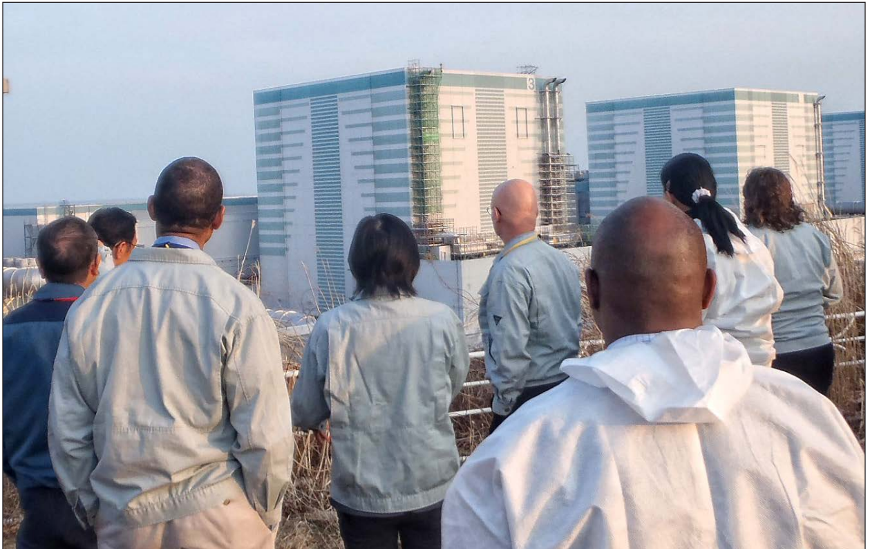
NRC Team looking at Units 3, 2, and 1 of the Fukushima Daini Nuclear Power Site.
