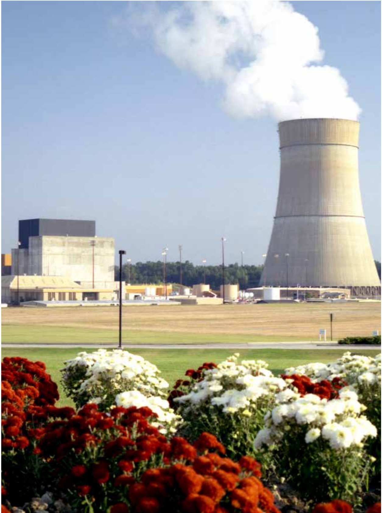
Grand Gulf nuclear power station. Photo courtesy Entergy-nuclear
