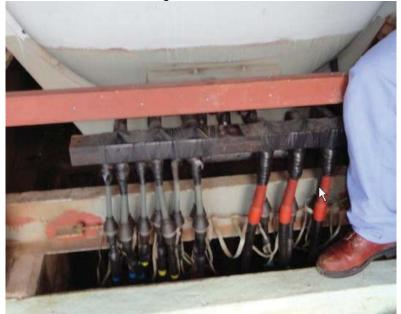
Emergency Diesel Generator output cables (Plant safety related DG's). Conceptual, other connection options are being evaluated.
