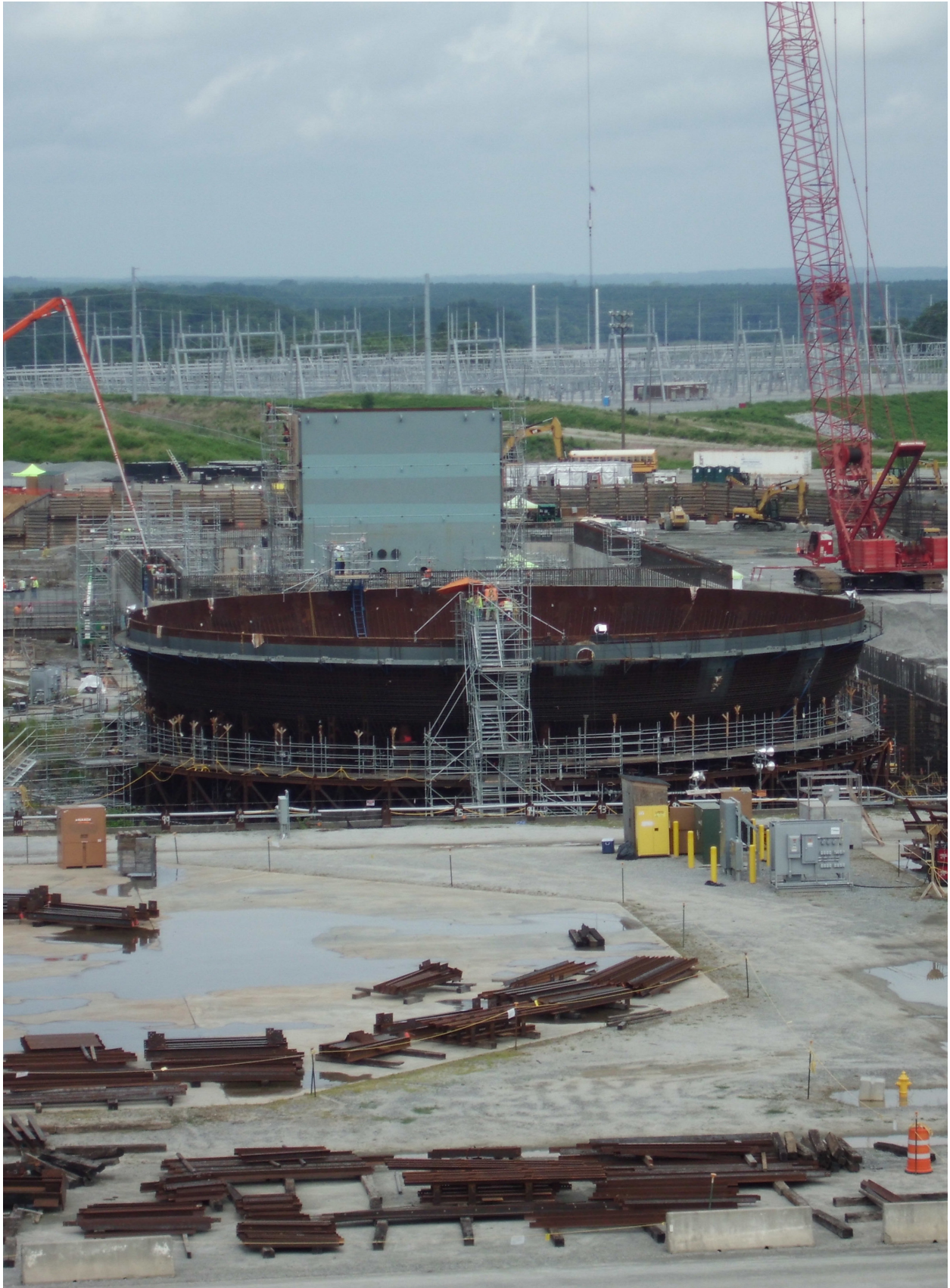
Construction progress at V.C. Summer Unit 3. Photo courtesy of David Failla.
