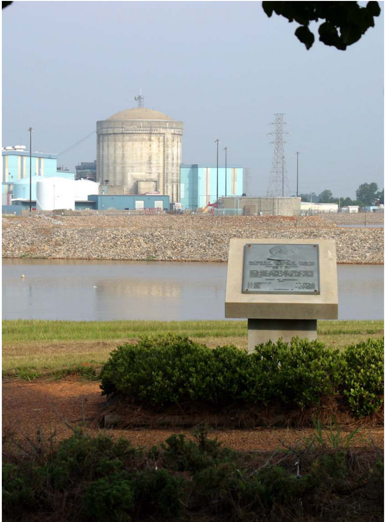
Virgil C. Summer nuclear power station. Photo courtesy of South Carolina Electric & Gas Company
