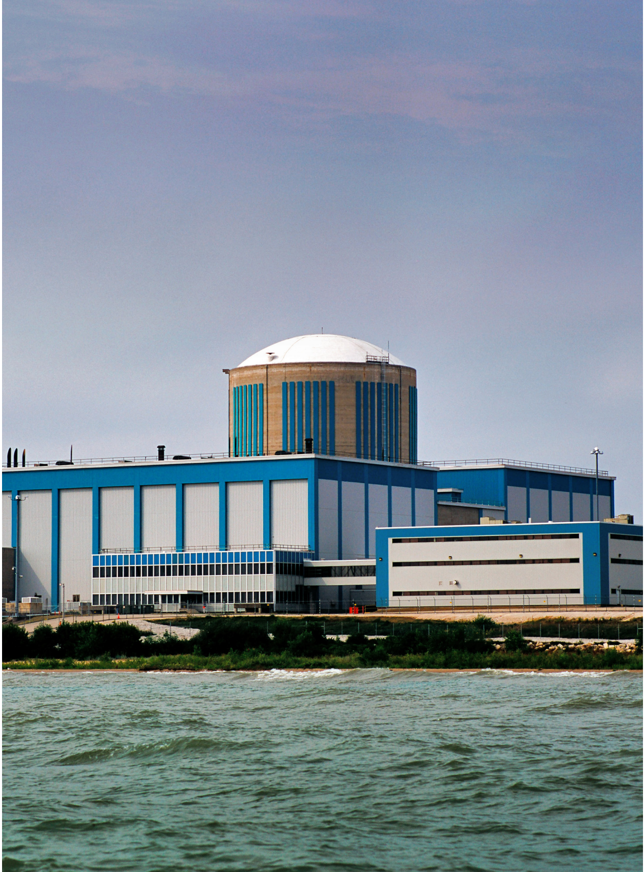
Keewaunee nuclear power station. Photo courtesy of Dominion Power.
