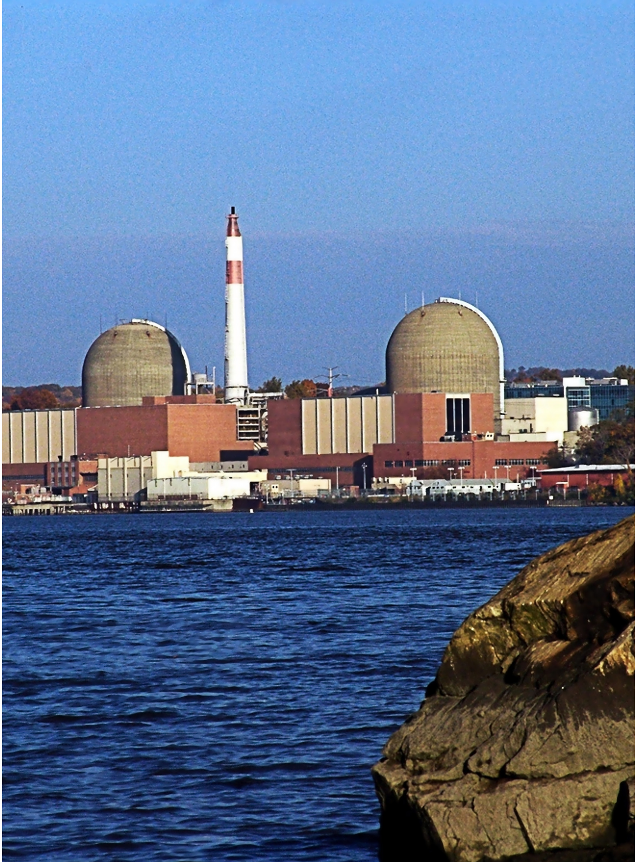
Indian Point nuclear power station. Photo courtesy of Entergy Nuclear Generation Co.
