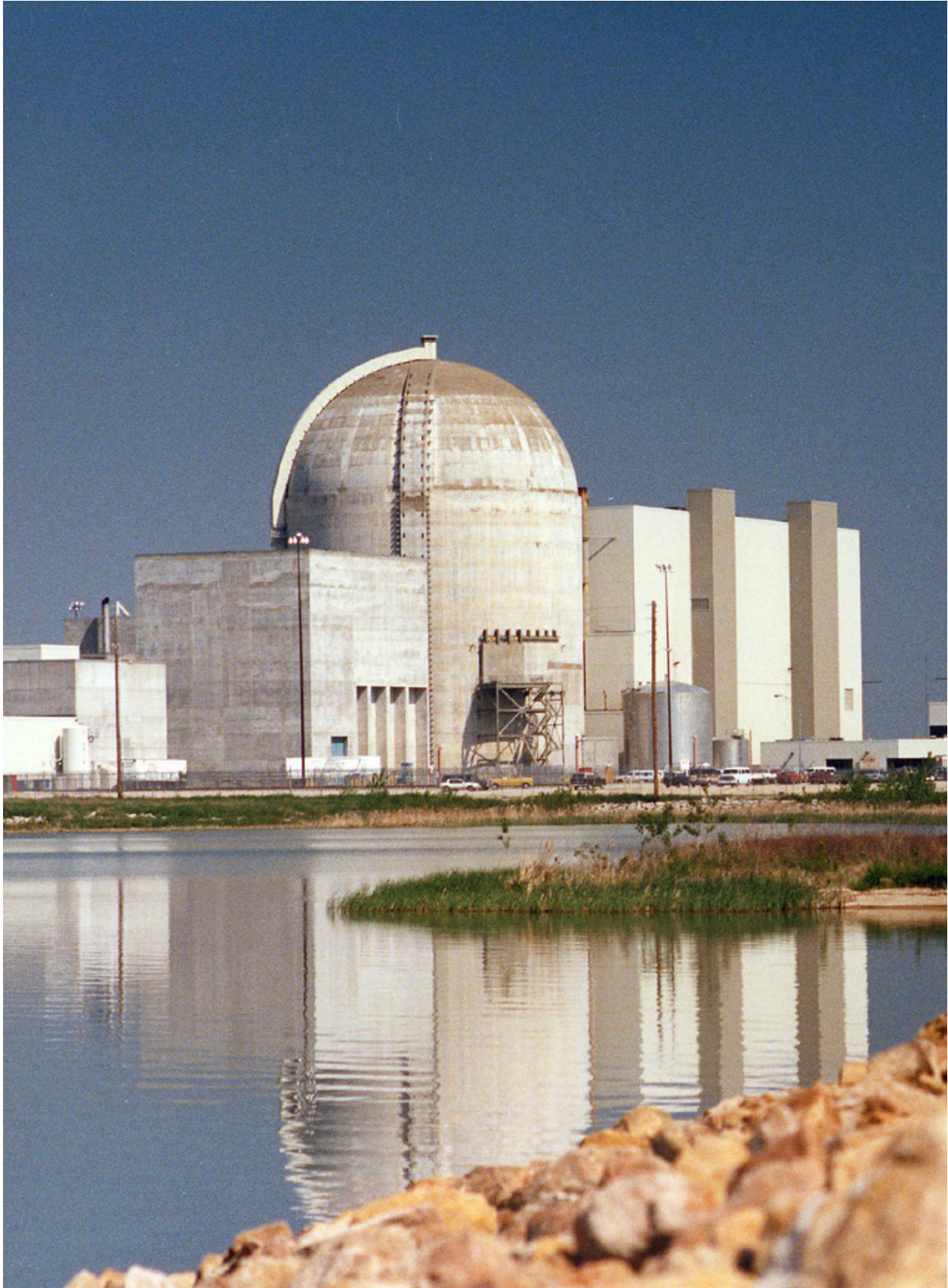
Wolf Creek nuclear power station. Photo courtesy of Westar Energy
