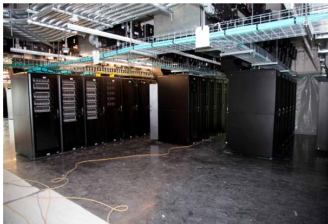
New Data Center Construction in Progress. Source: NRC
