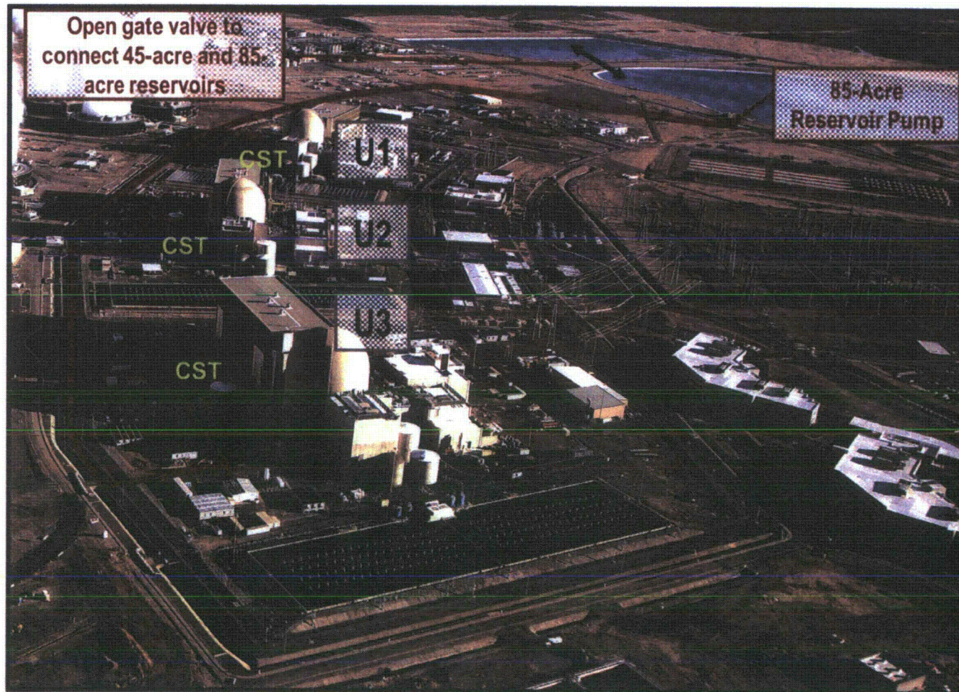
Figure 3-15: CST Makeup Pumping from the Reservoirs
