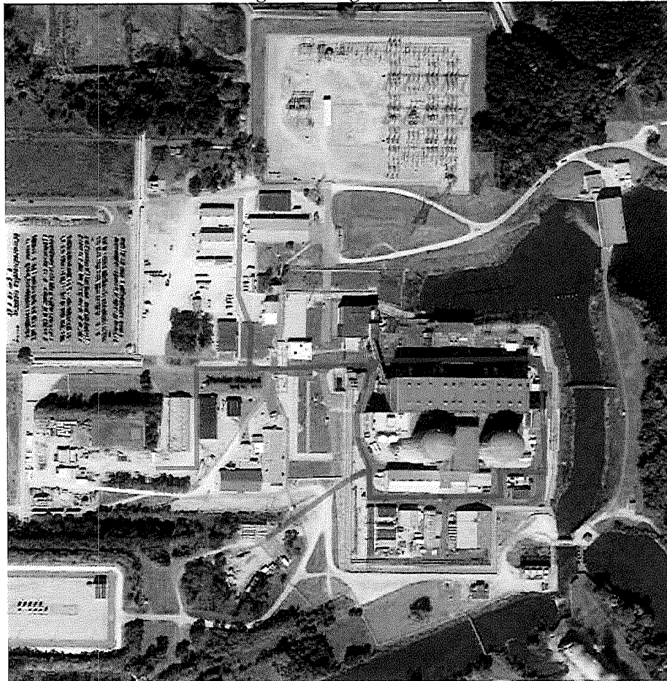
Figure 2 - On-Site Equipment Deployment Routes (identified pathways are preliminary and will be further evaluated during final design and implementation)
