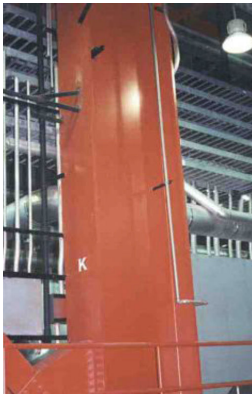
Figure F-3. Typical steel column in the turbine building.
