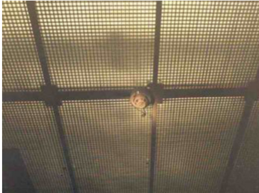
Figure A-3. Photograph of a typical open-grate ceiling.
