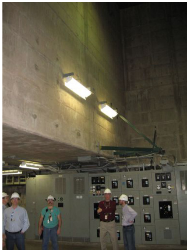
Figure D-3. View of the high ceiling space.
