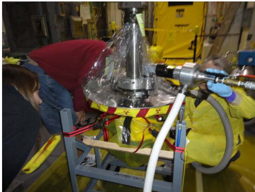
Figure 2.6 Cutting of Nozzle 63 Penetration Tube
