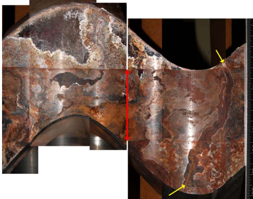
Figure 7.2 RPV Head Surface. The red line marks the span of the interference fit region and the two yellow arrows identify the main leak path.
