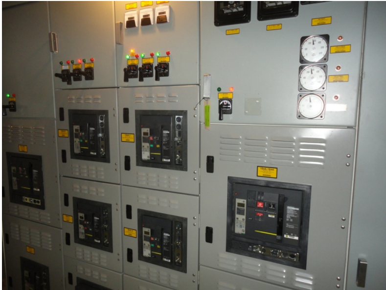
Restored Switchgear 1B4A
