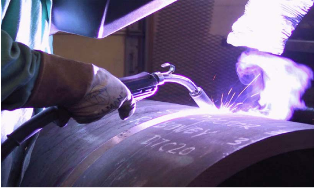
Figure A.10 Welding Root Pass with MIG
