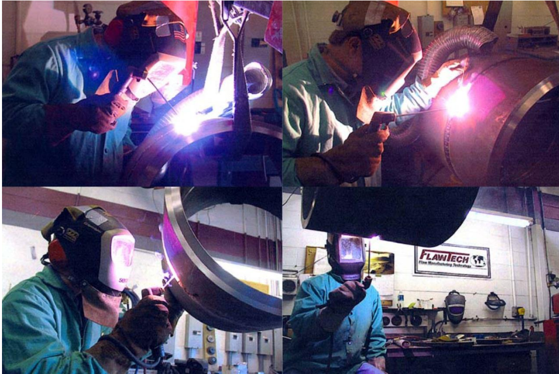
Figure 5.9 Field-like Welding on Horizontally Oriented Pipe Segments (photo courtesy of FlawTech Inc.)
