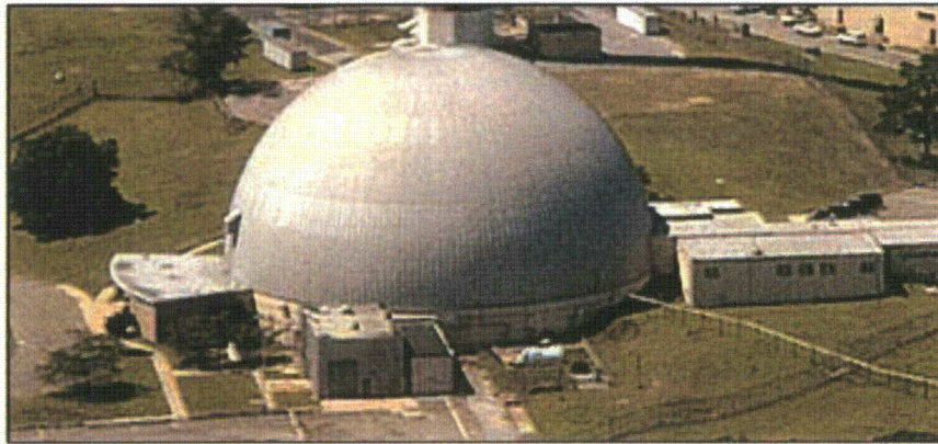
Figure 1-4: High Flux Beam Reactor (HFBR); (DOE, 2009)
