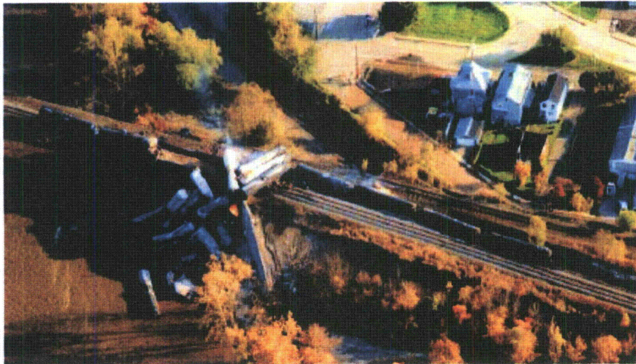
Figure 3-2. Photograph of Derailment, New Brighton, Pennsylvania, October 20, 2006. This Image is From National Transportation Safety Board RAR-08/02.
