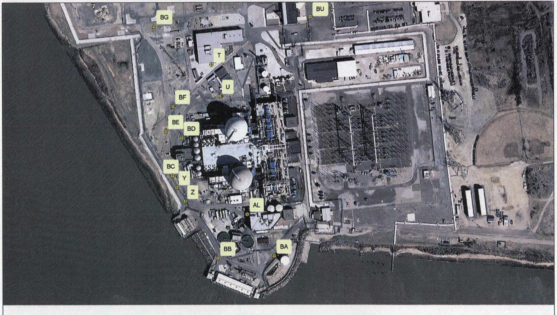
Figure 2 Salem RGPP Monitoring Well Locations
