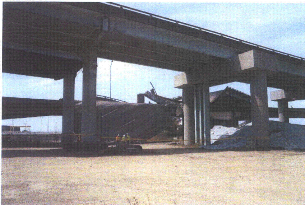
Figure 1-4. Post Fire Ground View of Collapsed Section of Interstate-580 California Department of Transportation (2007a)
