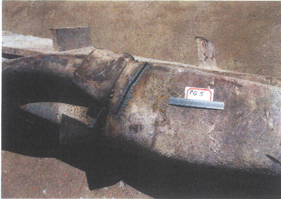
Figure 2-19. Photograph of Plate Girder 5 and Sample NRC 3
