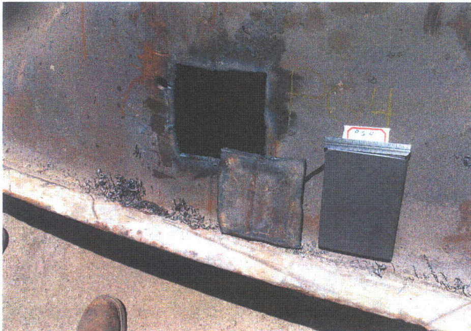
Figure 2-18. Photograph of Plate Girder 4 and Sample NRC 2
