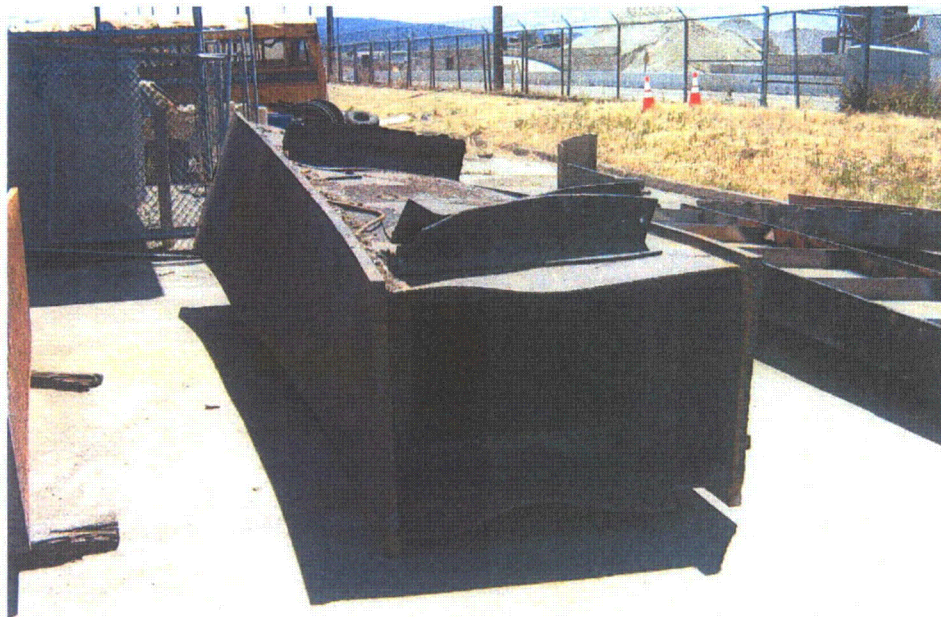
Figure 2-12. Photograph at the California Department of Transportation Storage Yard Showing Box Beam Cap Section 8
