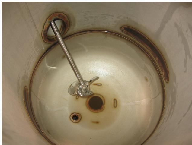
Figure 4: Debris Addition Tank Stirrer
