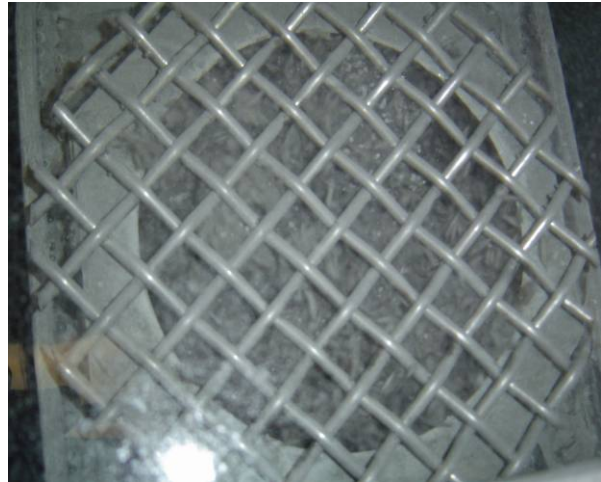
Figure 8: Wire Mesh Placed Over Chimney
