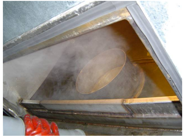
Figure 16: Internal View of Large-Scale Tank
