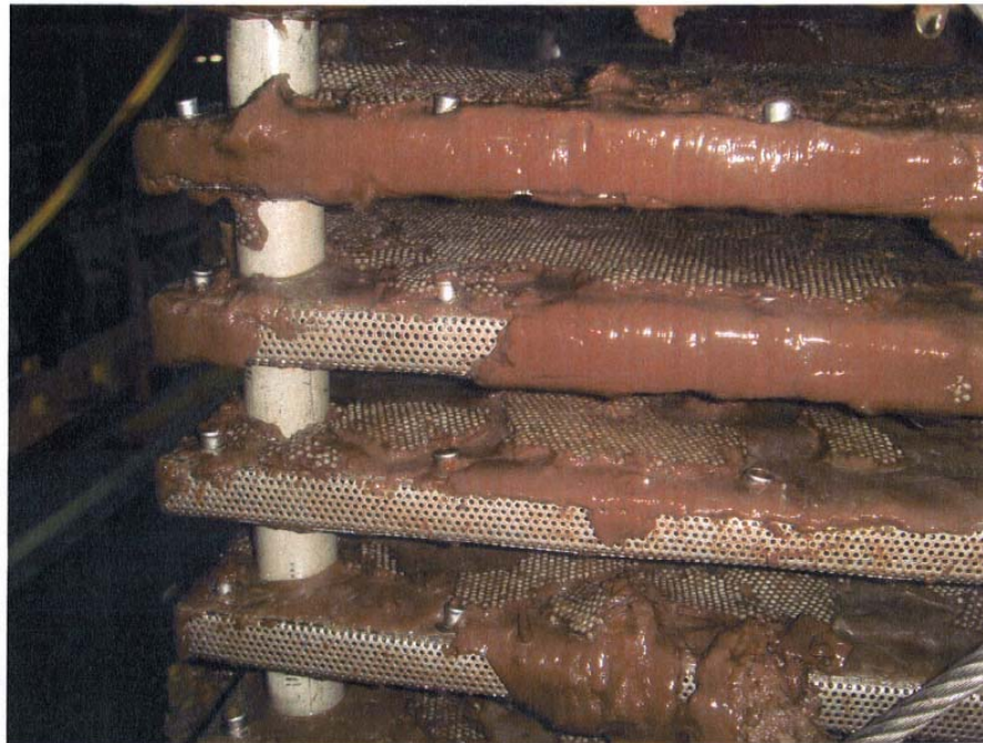
Figure 1. Evidence of Thin-Bed Debris Accumulation
