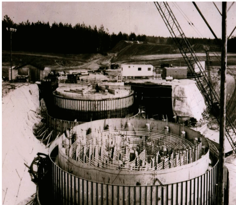
Figure 13: Tanks for liquid HLW storage under construction at the BNFP facility
