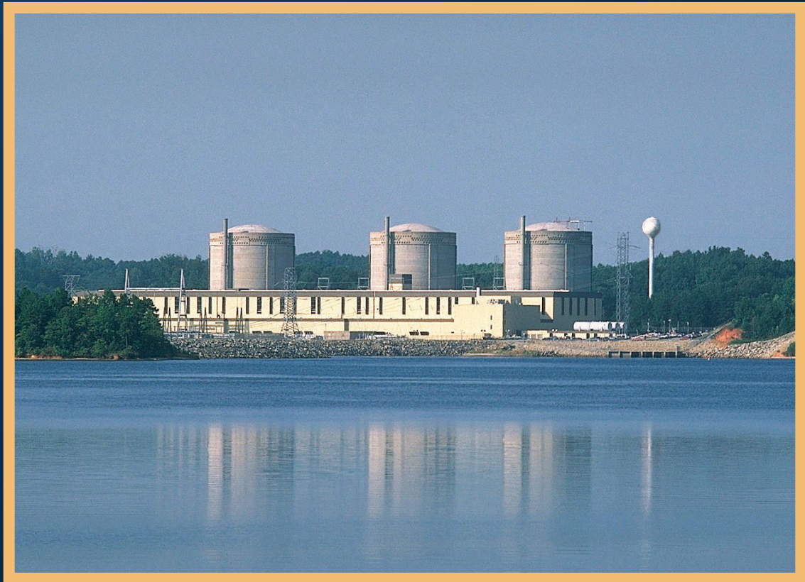
The Oconee nuclear station is located in Seneca, SC.
