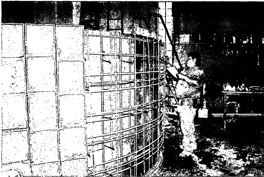
Figure 5. Strands and bars placed inside the form.
