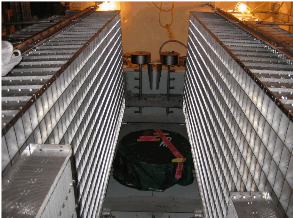
Figure 1 ONS Unit 2 Reactor Building Emergency Sump During the Replacement Strainer Installation
