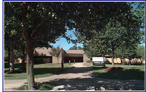
Duke Energy Corporation's Environmental Center
