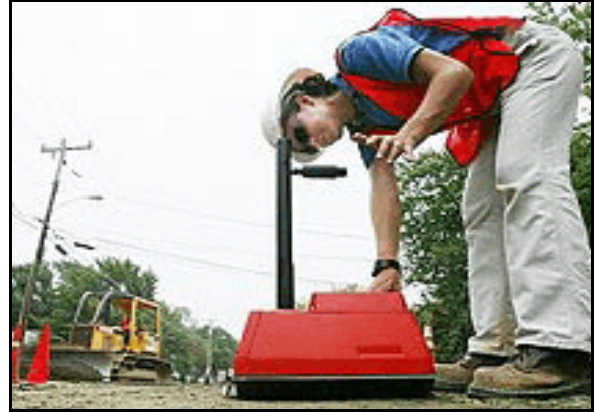
A typical moisture density gauge in use
