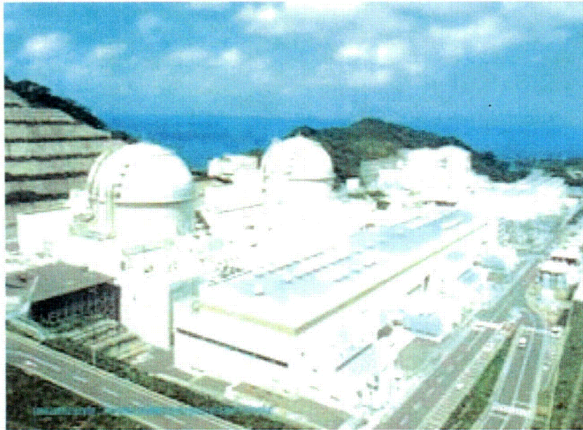
Figure 49 Ohi Nuclear Power Station, Ohi-cho, Fukui, Japan
