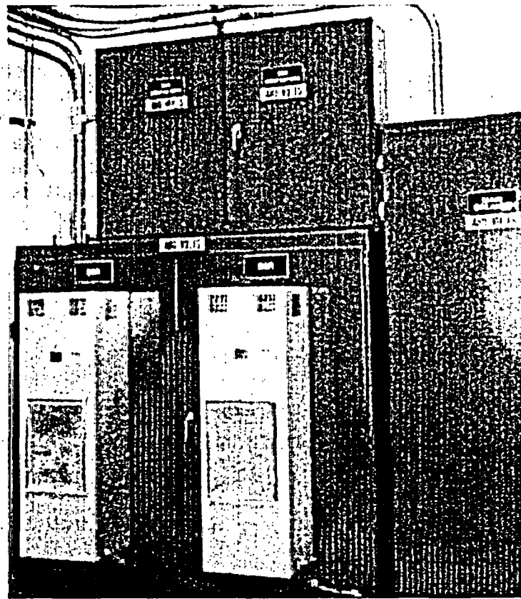
Figure 3.22. Photograph of the SCR Cabinet
