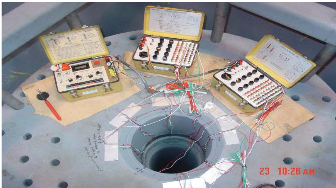
Illustration of the Installed Strain Gauges and the Strain Measuring Instrumentation at the Girard Site, Prior to MSIP Load Test
