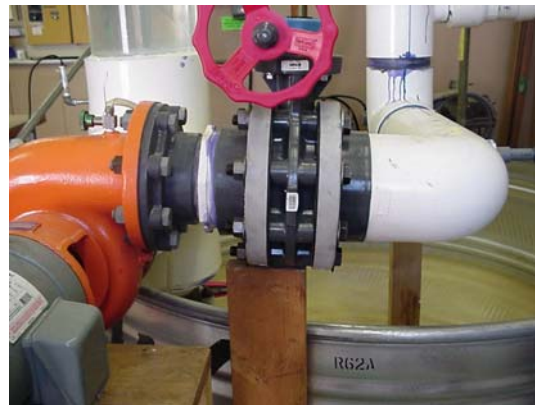
Figure A.12. Flow control valve adjacent to the loop pump.
