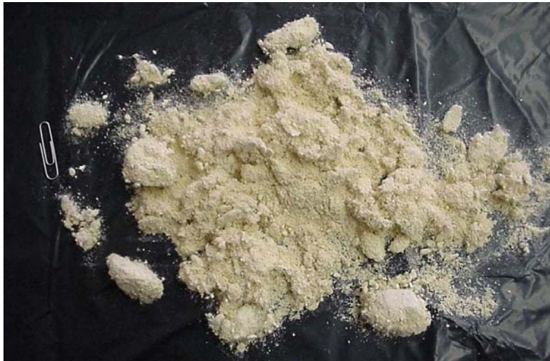
Figure C.2. Hand-crushed CaISil debris.
