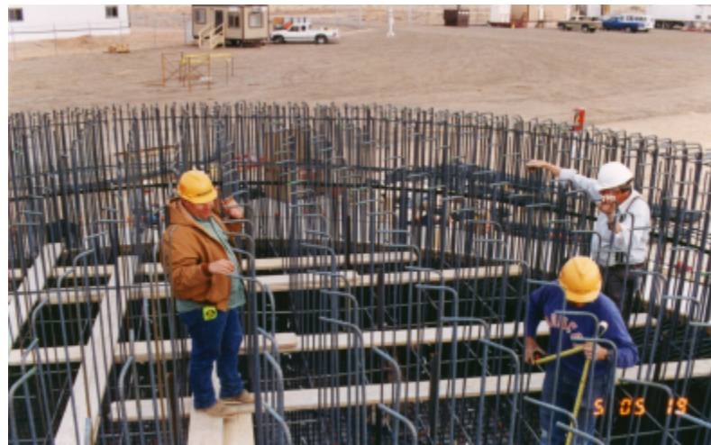
Figure 2.14 Basemat Bottom Bars and Vertical Ties
