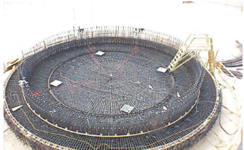
Figure 2.23 Basemat Top Rebar (F3) and Wall Dowels
