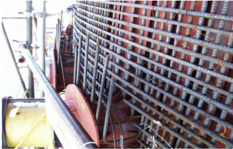
Figure 2.40 Inner Rebar at M/S Penetrations
