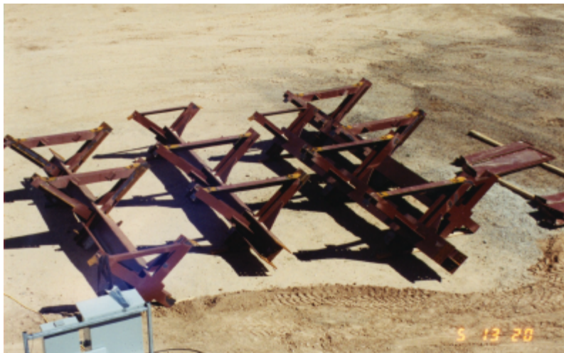
Figure 2.30 Instrumentation Frame Column 'Trees'
