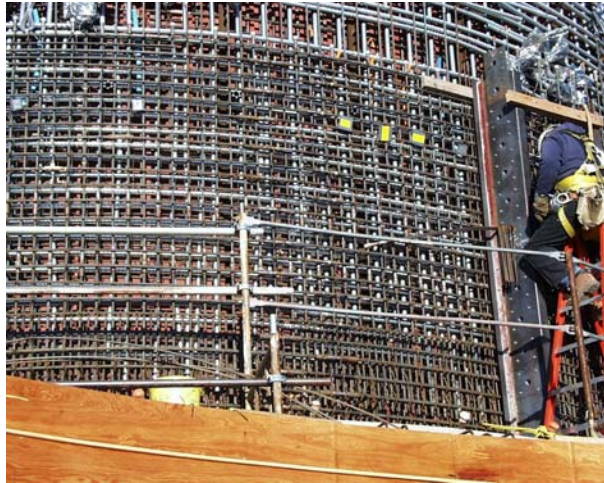
Figure 2.45 Outer Rebar for C1
