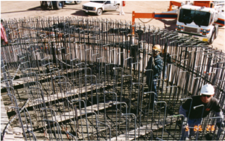
Figure 2.20 F2 Rebar Erection
