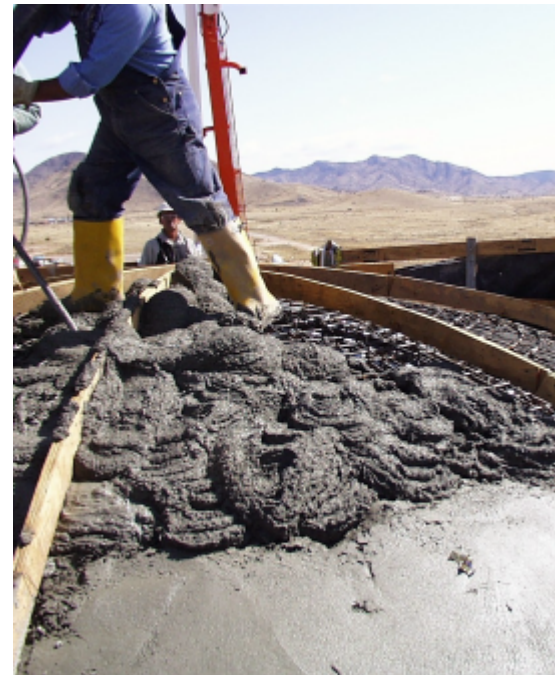
Figure 2.52 D3 Concrete Placement
