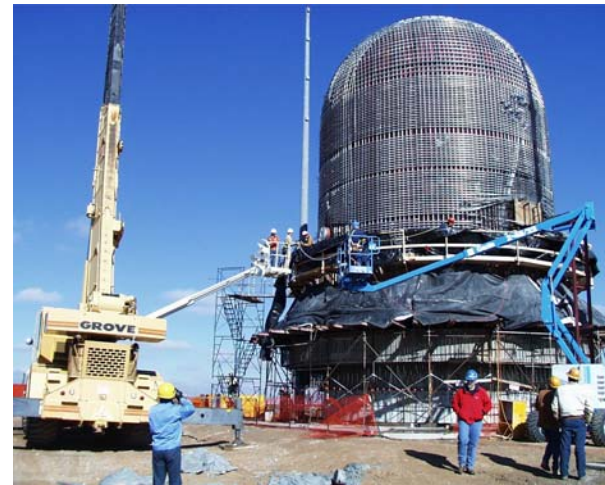
Figure 2.48 Installation of Instrumented Hoop Tendon.
