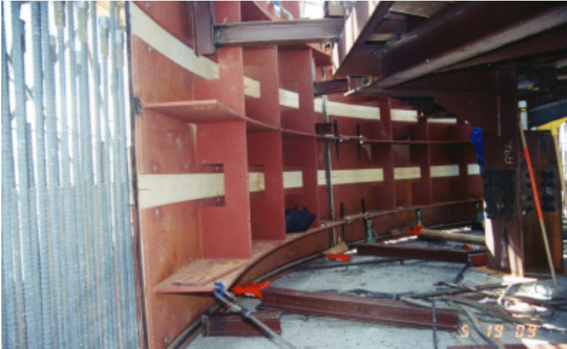
Figure 2.36 Liner Panels with Jigs
