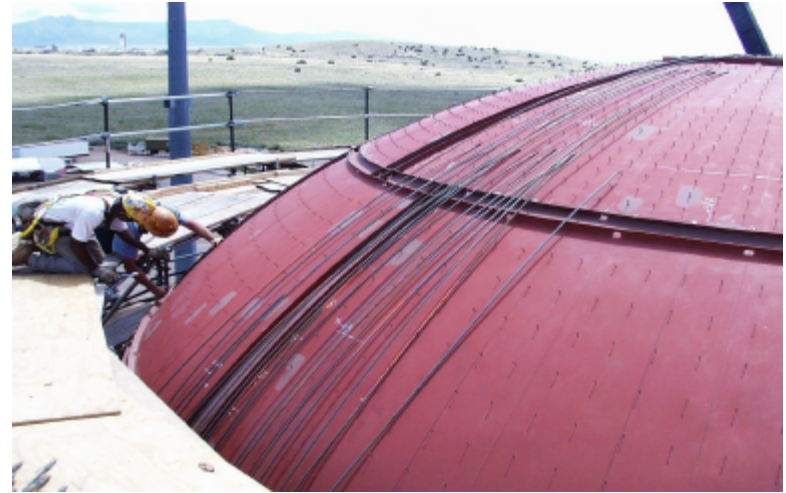
Figure 2.41 Installation of Inner Dome Rebar
