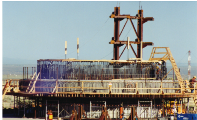
Figure 2.31 Instrumentation Frame Erection
