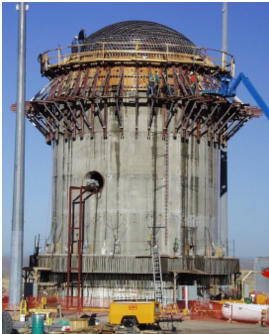
Figure 2.51 D1 Formwork Erection
