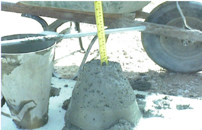
Figure 2.18 Measuring Concrete Slump
