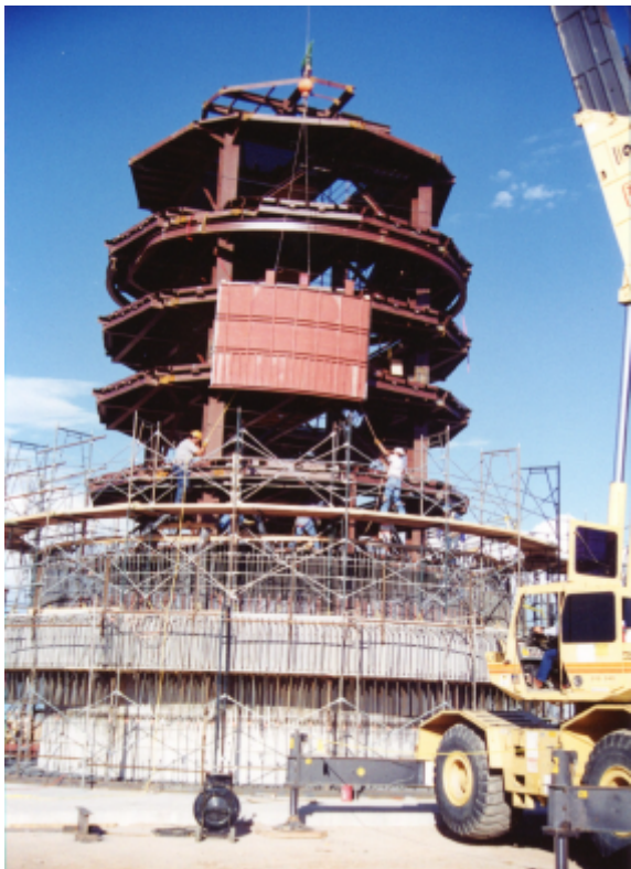
Figure 2.32 Instrument Frame Erection
