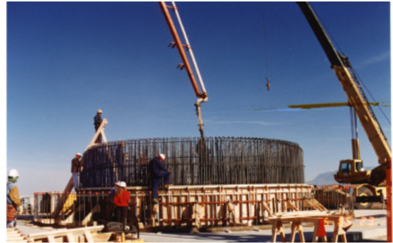
Figure 2.17 Placing F1 Concrete
