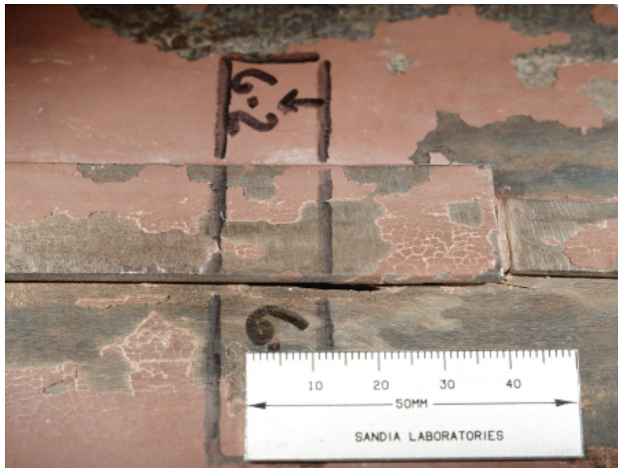
Figure 55. Details of inside (top) and outside (bottom) liner features in region of tear #6-2 metallographic cross-section (arrows begin at plane of section and indicate view direction).
