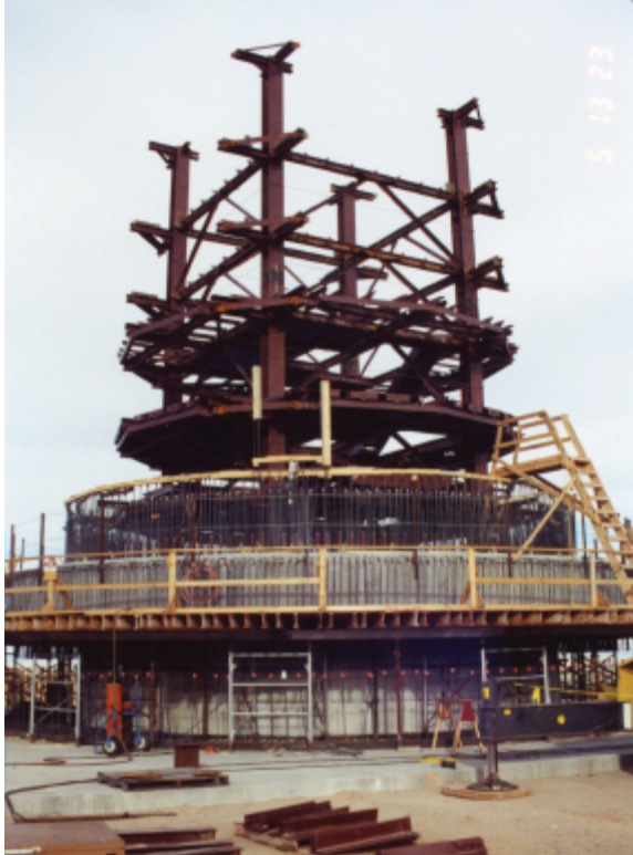
Figure 2.32 Instrument Frame Erection
