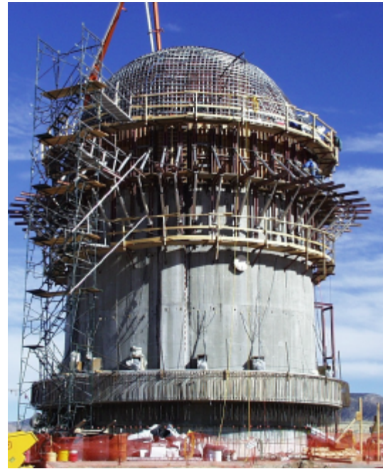
Figure 2.50 C4 Concrete Placement
