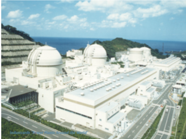
Figure 1.1. Ohi Nuclear Power Station, Ohi-cho, Fukui, Japan
