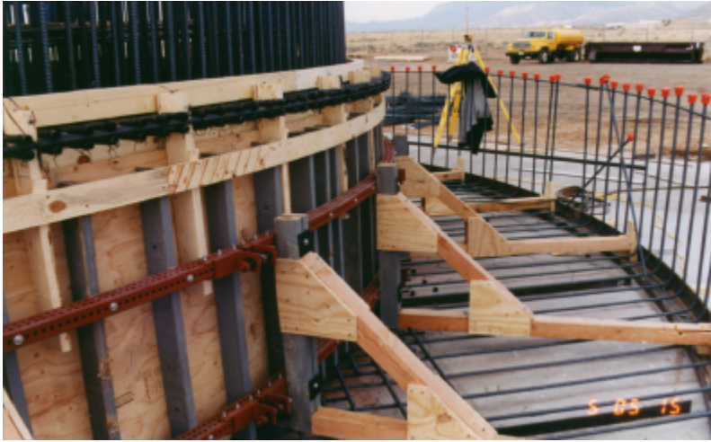
Figure 2.16 F1 Formwork
