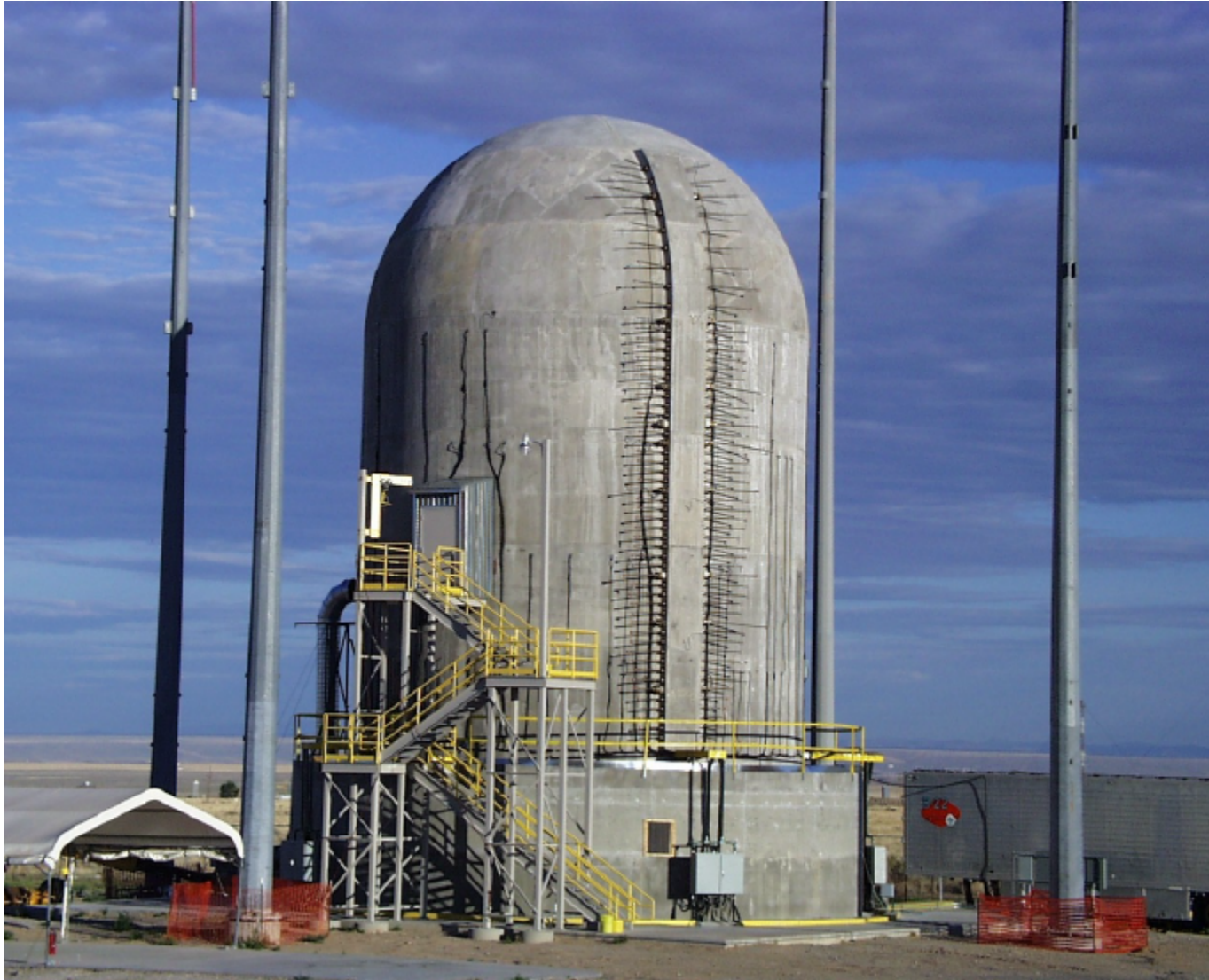
Figure 2.54 Completed PCCV Model
