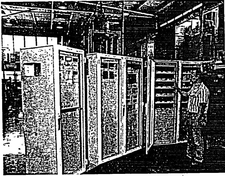
Figure 12. Facility control cabinets
