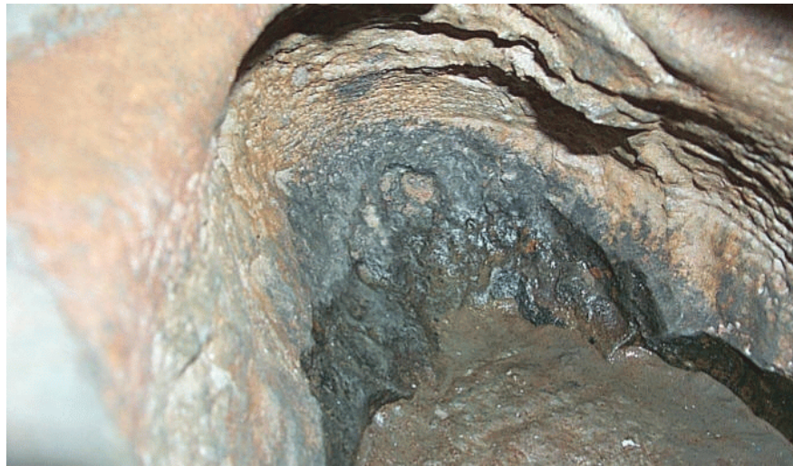
Close-Up View of Cavity
