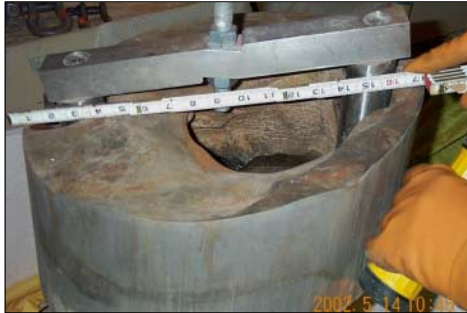
Nozzle #3 Area Cut Away From Reactor Head
